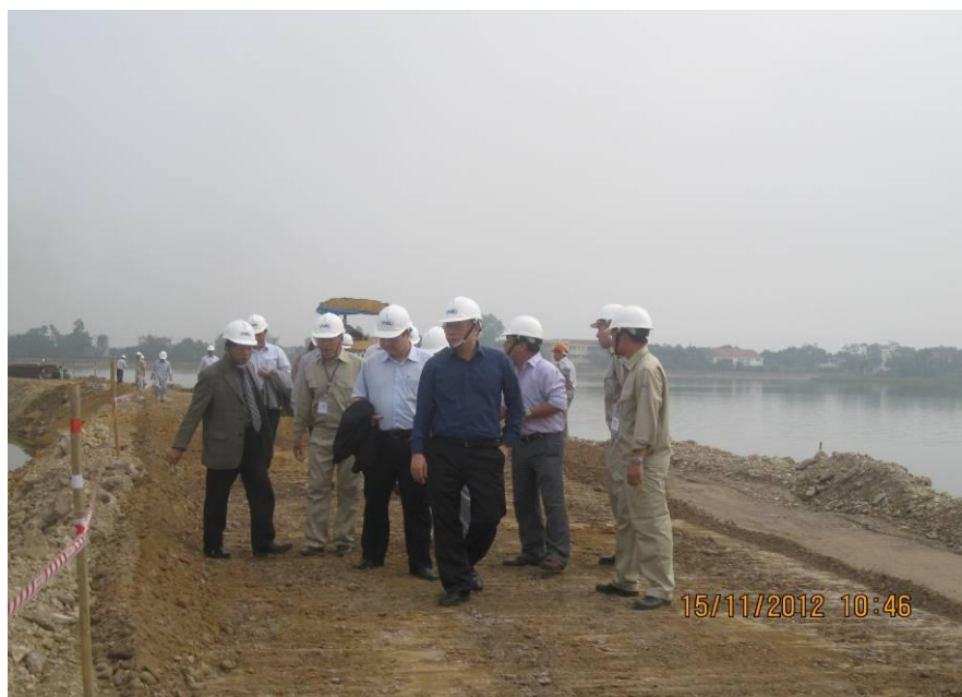
President of Vietnam Academy of Science and Technology visits construction site
