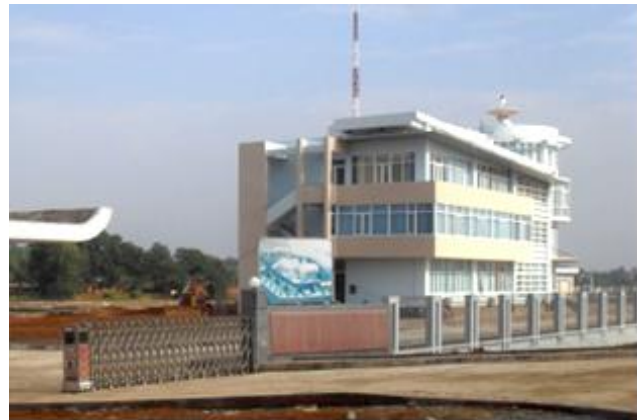
Sattellite control Station
