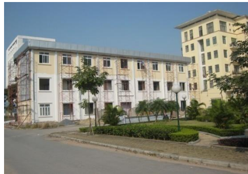
Improved building, A26, IAPSI
